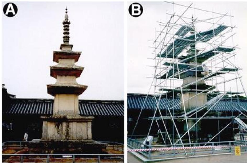
**Fig. 38.** A) The front view of Sukgatap pagoda. B) Detailed survey of the Sukgatap pagoda for stability (from Lee & Lee, 2007).
