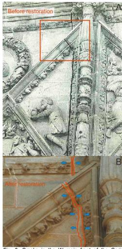
Fig. 3: Cracks in the W main front of the Coria's Cathedral. A) View before restoration; B) view after restoration in 2009.
