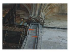
Fig. 7: Sinistral displacement of masonry blocks in the columns of the organ.
