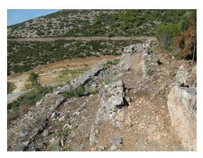
Fig. 4. Double channel of the Değirmendere aqueduct looking north. The lower channel is the older one and was partly demolished to build the upper channel on the right. Location shown in Figure 5.
