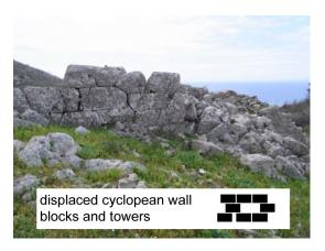
Fig. 7: Samicum, wall damage and tower collapse (Hellenistic period)
