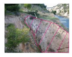
Fig.4: View of the secondary fault plane of the principal fault on the southern part of the Canal. It also created a landslide in the past.
