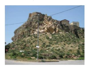
Fig. 3. Partial collapse of the easternmost point of Lorca's castle cliff. A detached rock-block produced damage in a near house.
