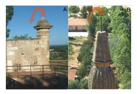
Fig. 5: A) Fall down of the balustrade's pinnacles in the south terrace of the Cathedral B) decapitated pinnacles in the north front of the Cathedral.
