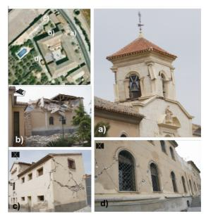
Fig. 4. Damage in the tower and main buildings of the Clarisas' Convent. (a) Destroyed tower, (b), collapsed roof of the main edifice, (c) and (d) X-fractures in the East and West sides of the annexed building.
