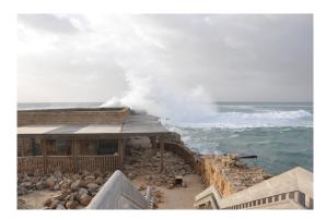
Fig. 2: December 15, 2010, Caesarea, Israel. Two days after height of major decadal storm. Rubble eroded from buildings and concrete slabs moved from the outer breakwater cover a structure on the harbour pier.
