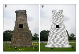
Fig. 4: (a) Overview of the damaged Cheomseongdae observatory in Gyeongju. (b) Sketch of southern part of Cheomseongdae.
