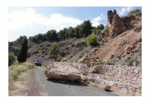
Fig. 2. Rock fall triggered by the Lorca earthquake and located at Las Estancias Sierra, southwestwardly of the epicentre location.
