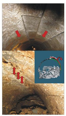
Fig.5: (Upper) Displacement of blocks in the vault of the western part of the Roman sewer. (Lower) Cracking of the vault in the eastern part of the sewer. In the bottom, the top of the filling of the sewer is still in place. The inset shows a cross-section of the point cloud when the sediment filling of the sewer was still in place. The green curve shows the original shape of the vault, the red line follows the rotated and displaced vault in the damaged area.
