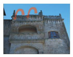
Fig. 4: Collapsed balustrade and pinnacles of the "Relics Balcony".
