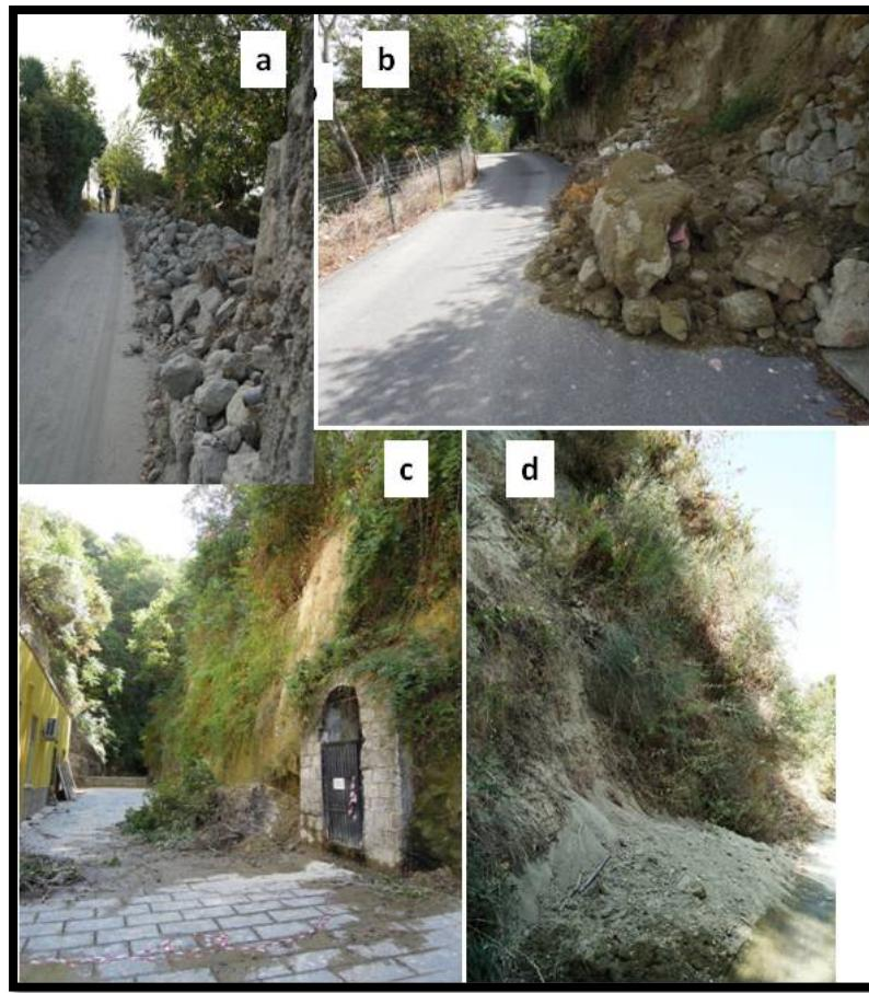
Picture 3: Collapse phenomena of drywalls at Casamicciola, in via dei Carri, (a), and in via Nizzola (b); Small landslides in volcanoclastic deposits in via Nizzola (c) and in via S. Barbara (d).
