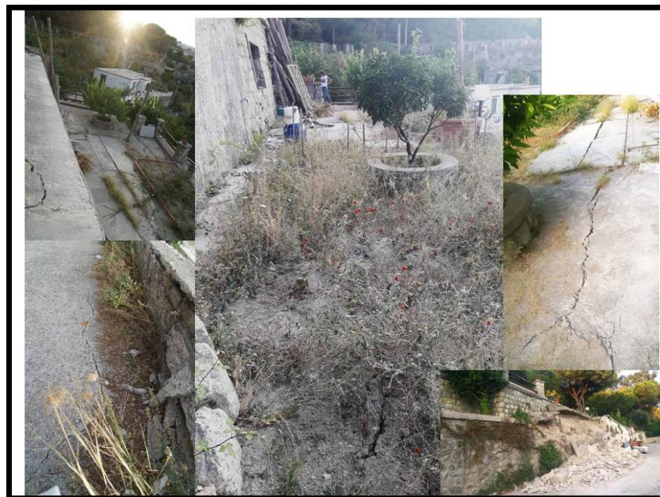
Picture 2: System of parallel surface coseismic fractures and drywall sliding in via Montecito (Casamicciola).
