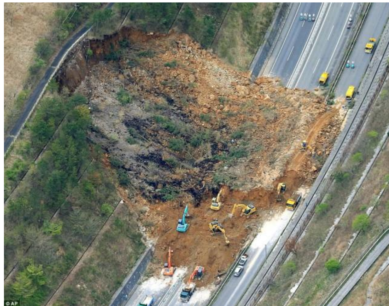
A major cutslope failure on the Oita Expressway, triggered by the Kumamoto Earthquake, via AP
