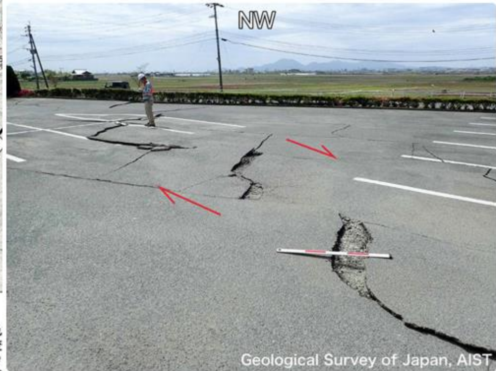
8-Akai village "mashiki townspeople rest of the house," parking lot to see is right-lateral displacement. Picture taken toward the northwest direction. Right-lateral displacement amount is about 40 ~ 50 cm. (2016 April 16 shooting)
