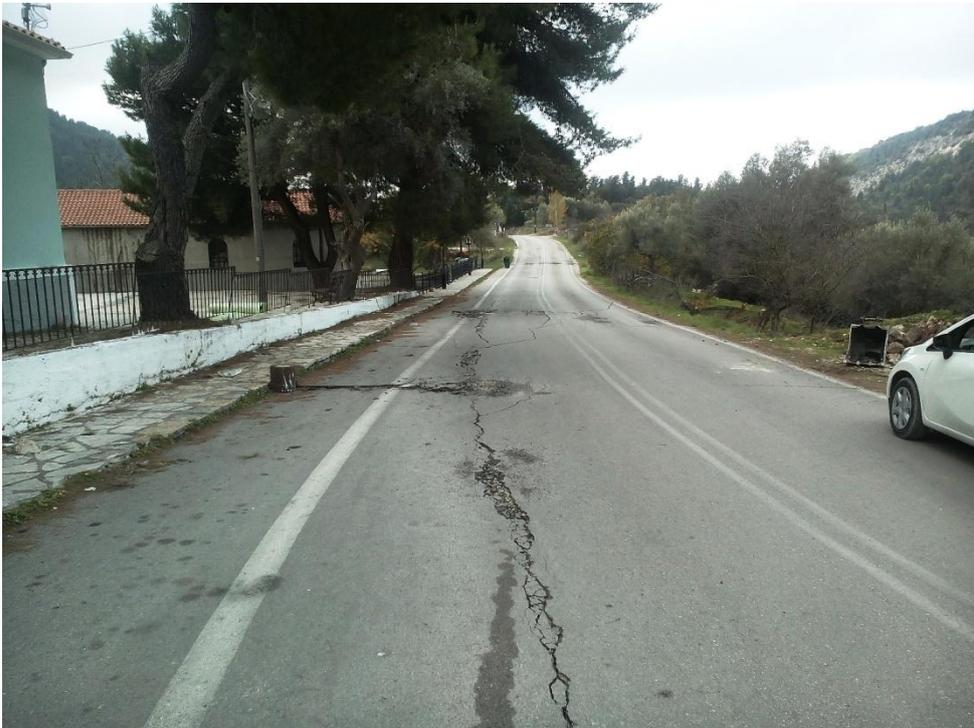
**Figure A2 .** Field photo of asphalt cracks along the road between Dragano and Athani villages. View to the south. Date photo was taken 20 Nov. 2015.
