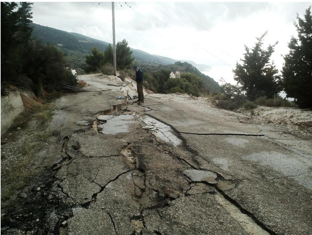
**Figure A7** Field photo of damaged road due to landslide at Platys Gialos beach. View to the south. Date photo was taken 21 Nov. 2015.
