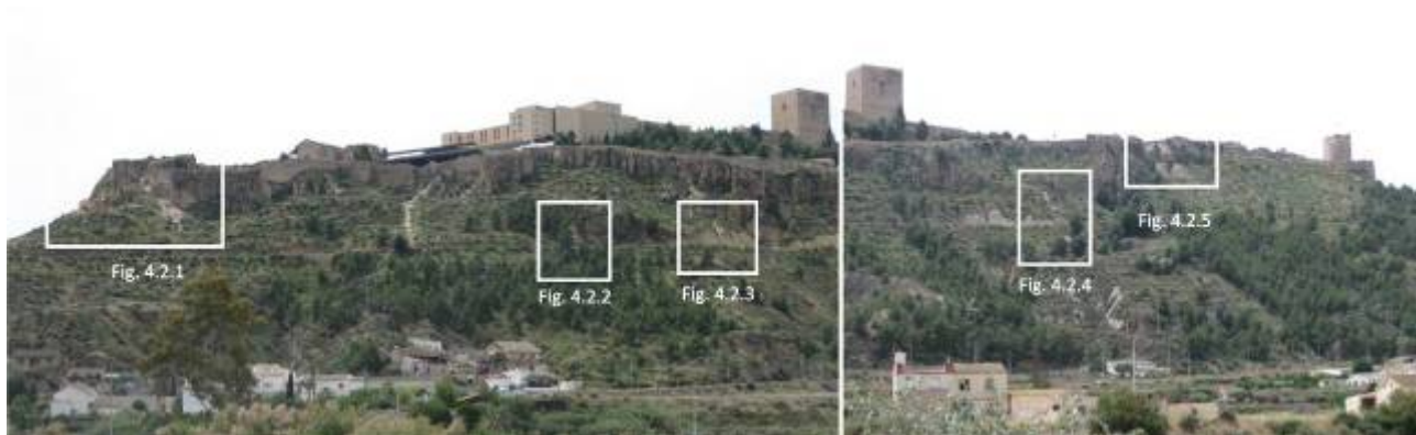
Figure 4.2.0: General view of the north slope of the Lorca's castle cliff. The most remarkable instabilities induced by the 11th May earthquake are identified.
