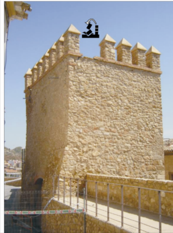
Figure 5.4: Damage in the battlements of the entrance of San Antonio (Tower of the old defensive wall of the Islamic Period).
