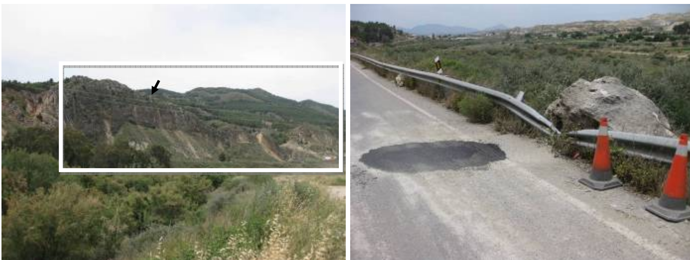
Figure 4.4.1b: Continuation of the Pantano de Puentes road towards the west. Along this road many instabilities were identified, although of a small size in general. Particularly remarkable are the rock blocks fallen from the ridge controlled by Las Viñas Fault (marked with an arrow). Picture on right shows a close-up of the damage produced by one of this rock blocks.
