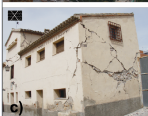
Figure 5.5: Damage in the tower and main buildings of the Clarisas' Convent.
