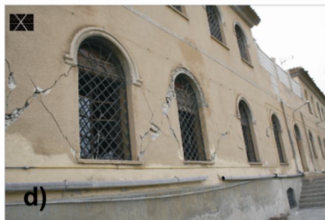
Figure 5.5: Damage in the tower and main buildings of the Clarisas' Convent.
