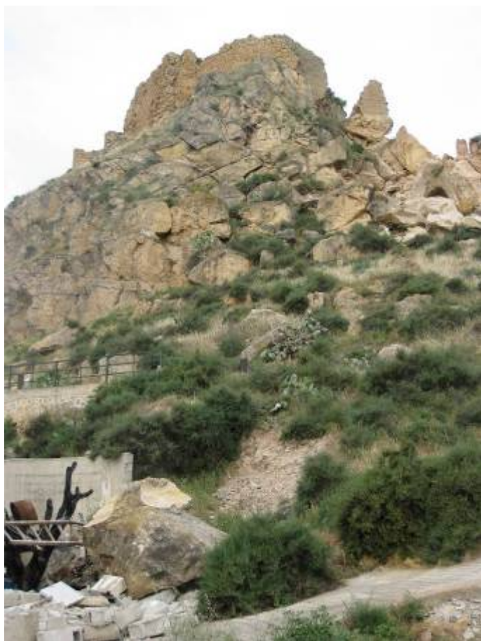
Figure 4.2.1b: View of south lateral of the easternmost point of the castle cliff and of the block that damaged a small wall of a house. The down-the-hill road pavement showed moderate damage at this point. It can be observed on the left the ending of the retaining wire mesh that stabilises the south face of the castle cliff.
