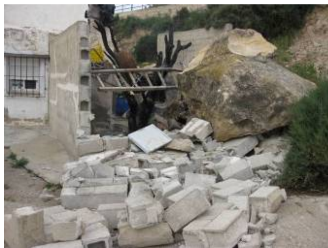
Figure 4.2.1c: Result of the impact on a wall made of concrete blocks enclosing the patio of a house from a rock detached from the easternmost point of the cliff.
