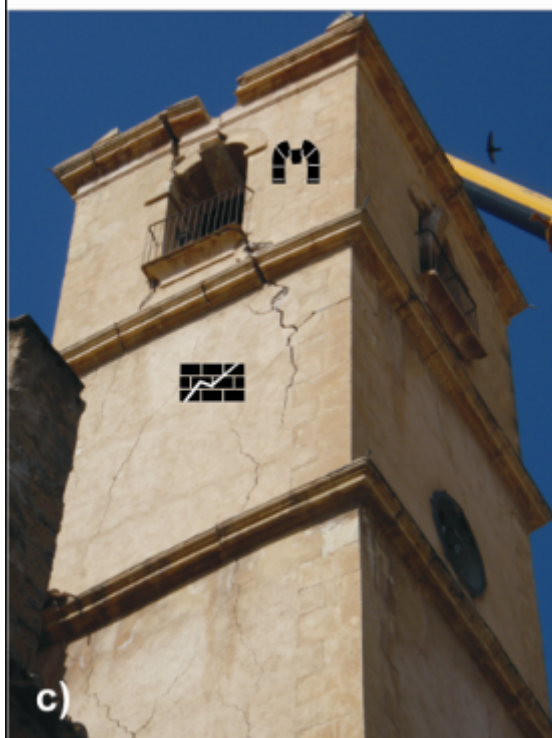
Figure 5.6: Damage in the San Francisco's Church.
