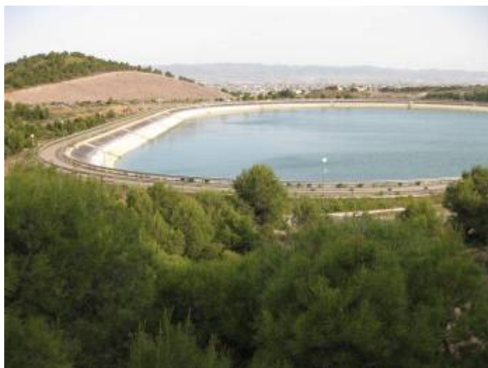
Figure 4.7: Irrigation pool situated nearby the epicentres of the 11 May earthquakes. Neither damage was observed in this area, nor instabilities on the talus on the background.
