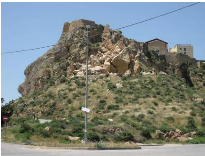
Figure 4.2.1a: Partial collapse of the easternmost point of Lorca's castle cliff. A detached rock-block produced damage in a near house (see Fig. 4.2.1c). Picture on right corresponds to the same place few years back (taken from the IGME seismic hazard study of Lorca, 1992).
