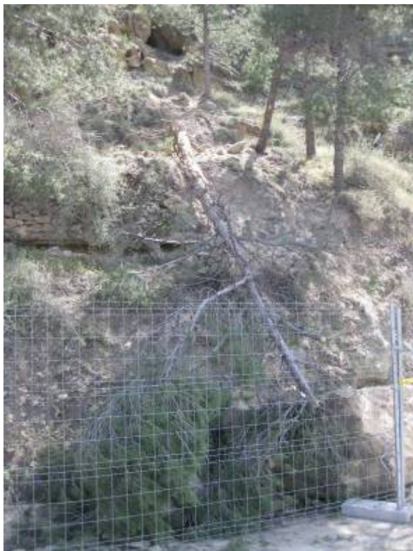
Figure 4.2.2: Small debris dragging a pine tree on the north talus of the up-the-hill road to the castle.
