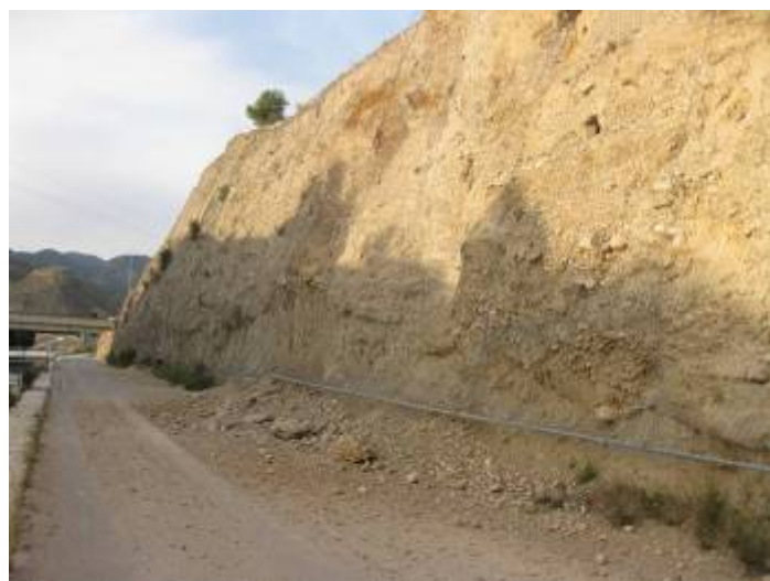
Figure 4.9: Shallow debris falls attributed to the May earthquakes on a service road of the Tajo-Segura canal.
